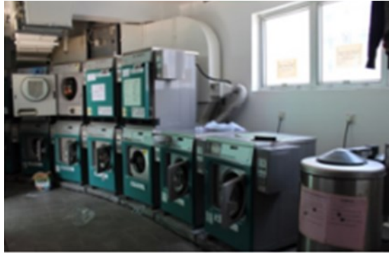
Laundry room at 10th floor.
